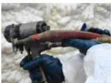
**Chemical Resistant Gloves:** Wear fabric gloves fully coated with nitrile, neoprene, butyl, or PVC. Alternatively, cotton gloves over disposable nitrile gloves may be used.
