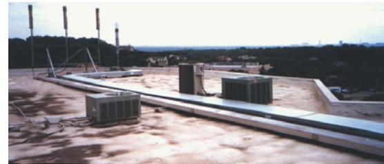
**Case Study 2:** An SPF roof was applied directly to a single-ply membrane; the expansion of SPF caused the roof surface to "mound up" between fasteners. The SPF was well adhered to the existing single-ply membrane but that membrane was only intermittently secured (mechanically fastened) to the roof deck. The result was an appearance failure (although roof traffic could have eventually caused other problems).
