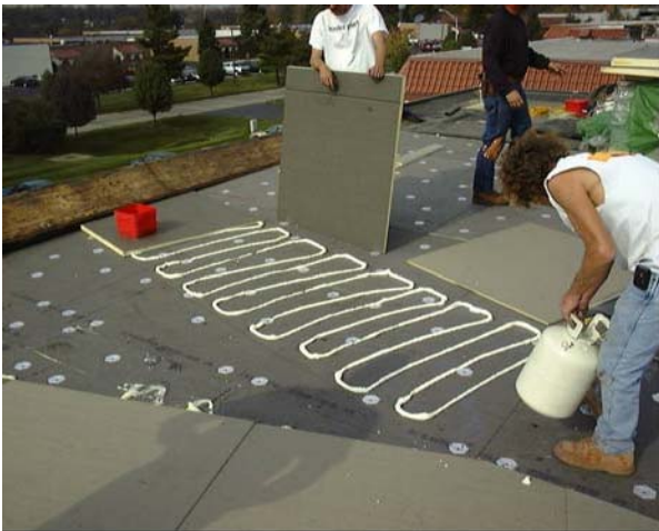
Figure 4: SPF Adhesive ribbon application.
