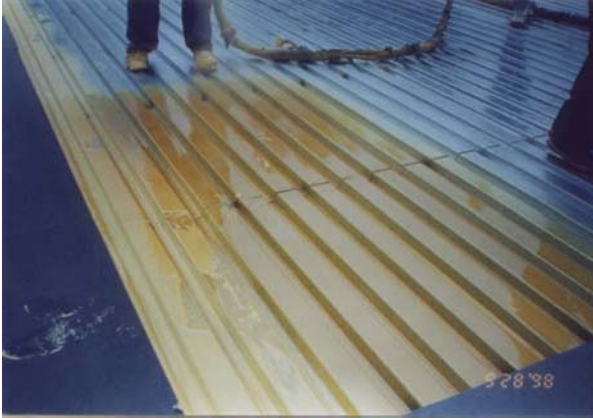
Figure 3: SPF Adhesive full coverage application.
